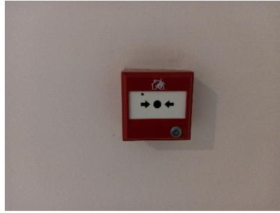
fire alarm manual station
