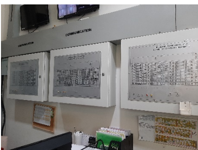
Graphic Annunciator Fire Alarm System
